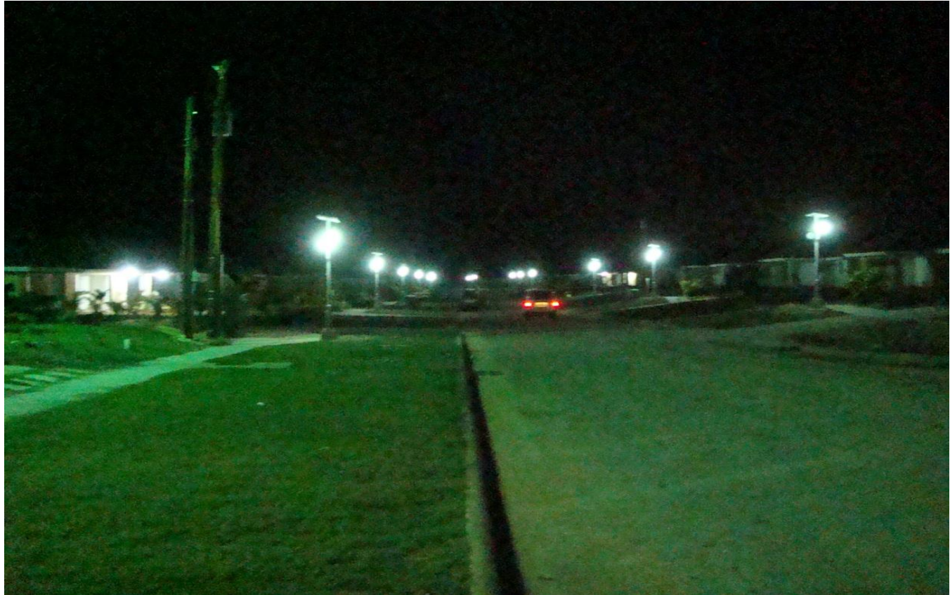
Richmond Housing Development in St. Ann – Streetlights in Phase 1
