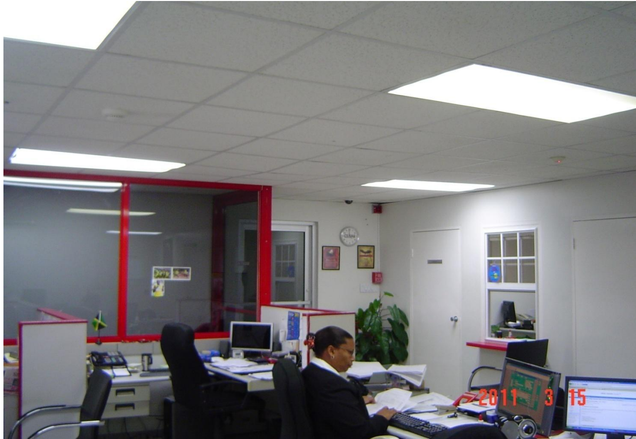
LED Lighting Installation at Hawkeye
