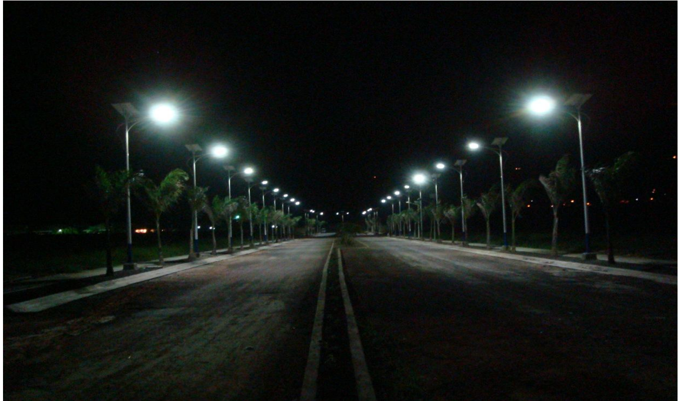
Richmond Housing Development in St. Ann – Streetlights at Entrance
